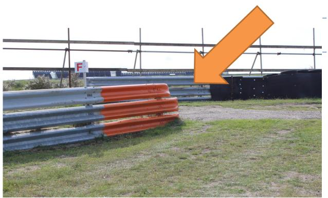
An orange armco means an opening in the guardrail.
